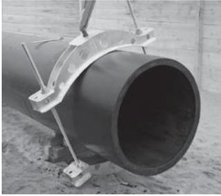
For rounding back HD-PE pipes.
